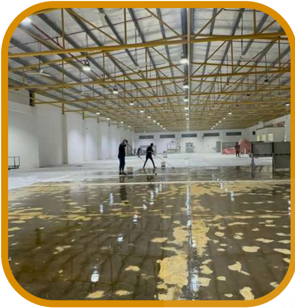
PRIMER APPLICATION PRIOR EPOXY COATING
