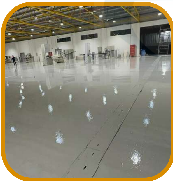
EPOXY COATING / PAINTING
